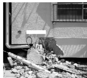
Fig. 2 Failure of beam-column joint
