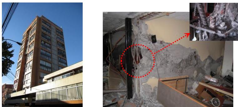
**Figure 1.** Damage of multi-story bearing wall without boundary columns at the 2010 Chile Earthquake
